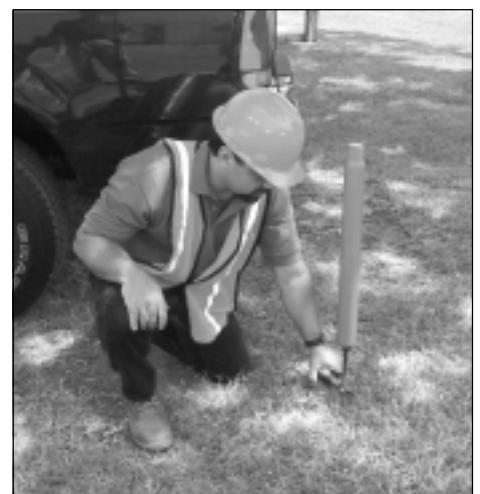
Temporary insulated ground for utility vehicle
