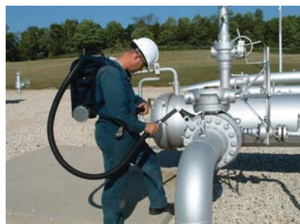
Technician measures valve grease fitting leak utilizing the Hi Flow Sampler.
